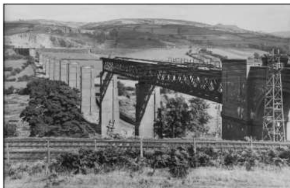
Llanbradach Viaduct during its demolition in 1937 - WRA Vol. VII No. 9
