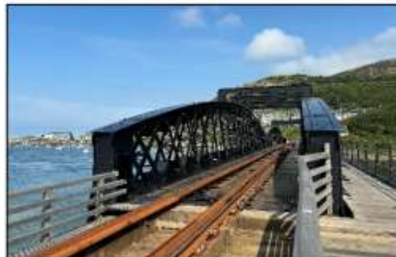
New main girders of Barmouth Bridge (2024) - WRA Vol. VII No. 10
